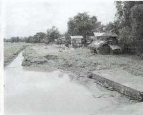
Pic3.2 The same barangay on the left after floodwaters had subsided.
