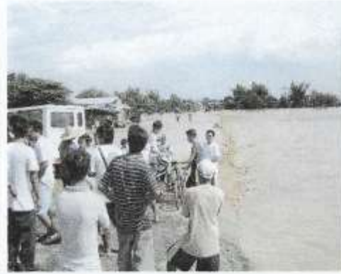
Pic 3.0 Pampanga River overflowed the Cabiao floodway at around 1000H of November 30, 2004.
