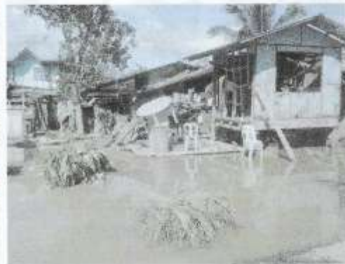
Pic 4.1 A still flooded Bgy. Magpapalayok in San Leonardo, N.E. The area suffered almost 3 floodings for the year 2004.
