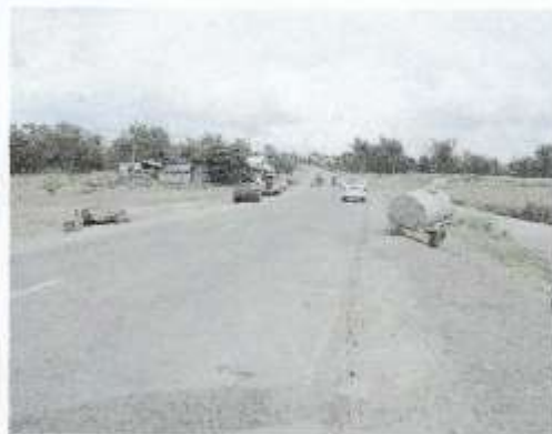
Pic 3.4 The GSO road several days after the flood event.
