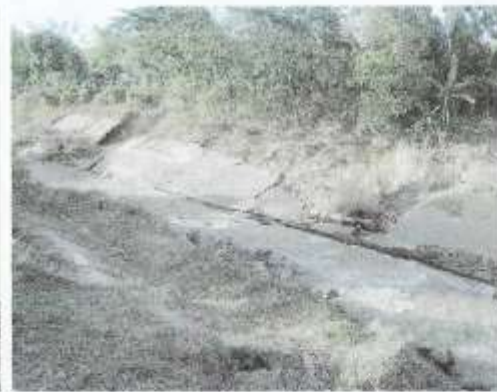
Pic 13.0 Scoured embankments along the Minatula River, between Sta. Rosa and Cabanatuan, N.E.
