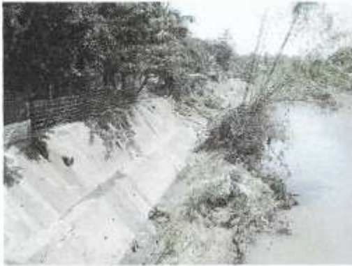
Pic 18.0 Eroded embankment as a result of flash floods along the San Miguel River near Poblacion of San Miguel in Bulacan.
