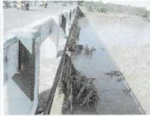
Pic 19.0 Debris brought about by floodwaters along Pampanga River at Jaen - San Isidro Bridge.
