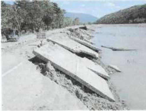
Pic 6.0 The Gabaldon - Laur road in Bato Ferry, Laur, N.E. was washed-out as a result of the overflowing of Coronel River.
