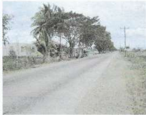
Pic 10.1 The same area on the left a month after the flooding.
