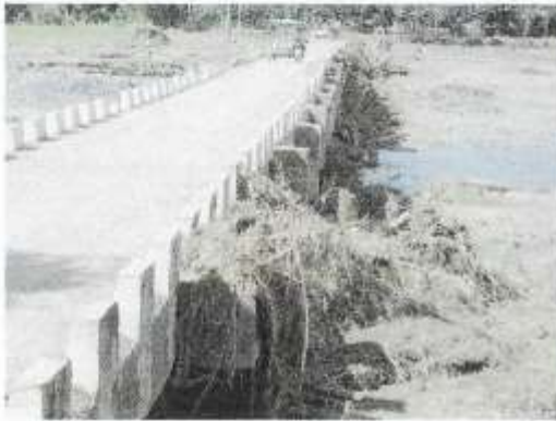
Pic 15.0 More than a meter of floodwaters from Chico River overflowed this bridge in Bgy. Papaya, Gen. Tinio, N.E.
