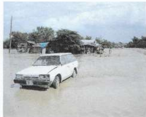
Pic 3.6 About 300 meters of 0.5 m deep of floodwaters covered a stretch of the GSO road in Cabiao, Nueva Ecija.
