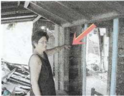
Pic. 5.0 Maximum flood depth of about 1.3 m attained in Barangay San Anton, San Leonardo, Nueva Ecija.
