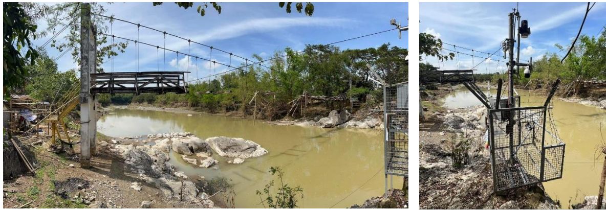
(Pic 11, Top L) The hanging bridge walk over Madlum River in San Miguel, Bulacan was washed out as floodwaters spawned by Karding rose to more than 4 to 5 meters in the area. (Pic 12, Top R) A monitoring station of the Bulacan-PDRRMO was also damaged during the event as floodwaters swept through the said station as high as to the station's utility box. (Photos shared by Bulacan-PDRRMO)
