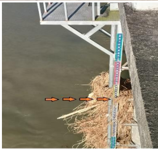
(Pic 35, Above) Pampanga River at San Agustin Bridge in Arayat just a few hours before cresting at 8.26 m at 1900H, Sept 26 (photo taken at 1100H, Sept 26 at a telemetry reading of 7.98 m) (Pic 36, Far L) Coronel River at Bangkerohan Bridge in Palayan City at an estimated gage of 3.40 m (1646H, Sept 26); (Pic 37, L) Staff gage at Peñaranda Bridge with debris still clinging at just below the 6.0 m mark (1628H, Oct 06)
