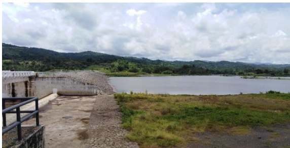
(Pic 61, L) Upper Tabuating Dam, somewhere in Gen Tiño in NE and still under NIA-UPRIIS, had a maximum dam overflow spillage of only 1.80 cumecs on 1200H of Oct 30. This dam is a relatively quite small water impounding and overflow reservoir and mainly for irrigation purpose only with just having a drainage area of 18.38 km 2 .
