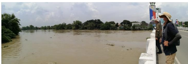
(Pic 33, L) River velocity measurements of the Pampanga River were carried-out at the San Luis Bridge in the town of San Luis in Pampanga as of 1235H, Sept 29.
