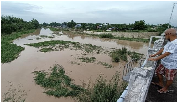
(Pic 50, Left picture) Abacan River as seen downstream from the Mexico Bridge II in Sto. Rosario, Mexico, Pampanga a day after Karding's passage (1011H, Sept 26) showing no definite signs of a relatively high flow (grasses within the channel are still standing).
