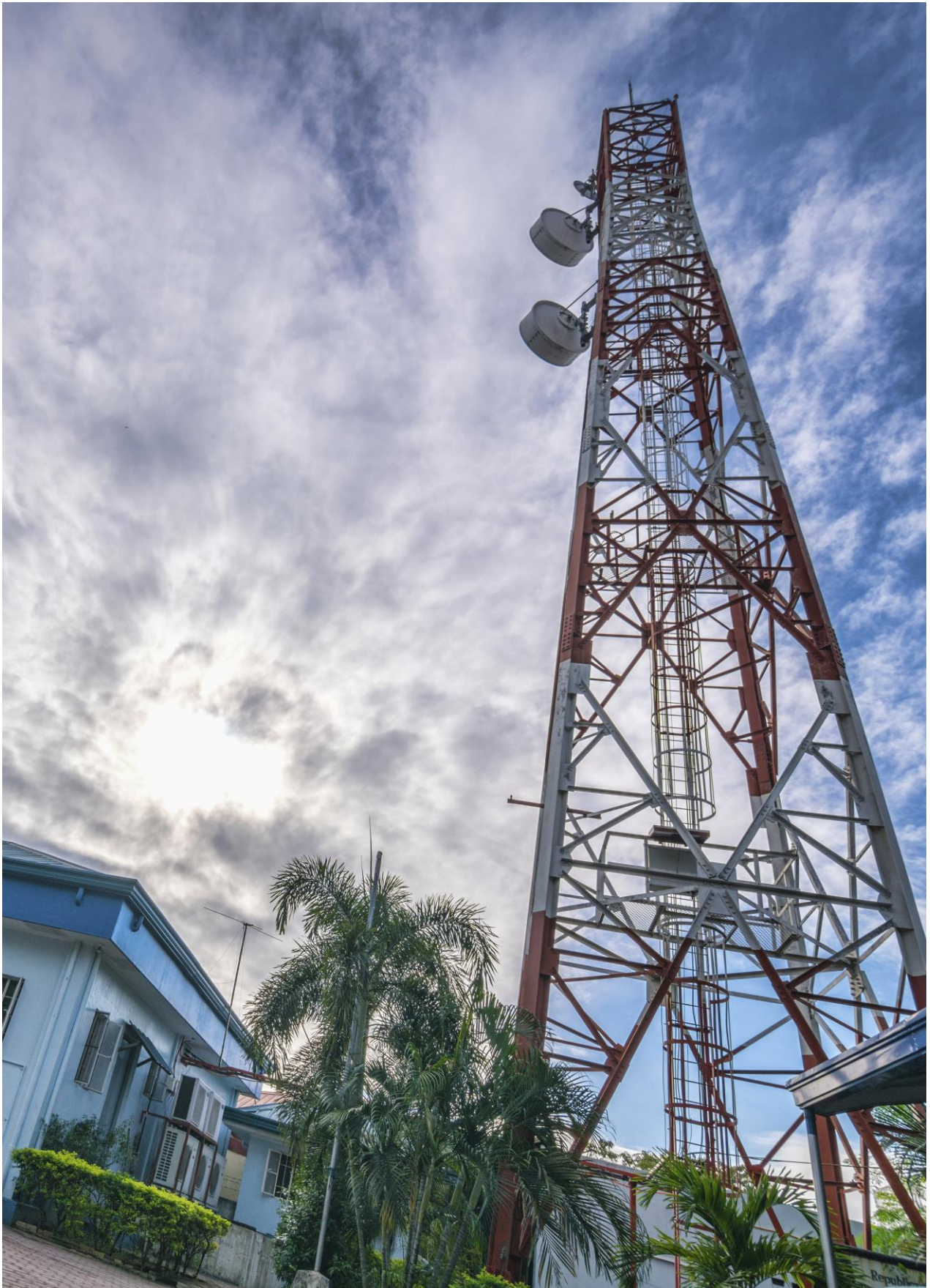
The PRFFWC Telemetry Tower located in the City of San Fernando, Province of Pampanga.
