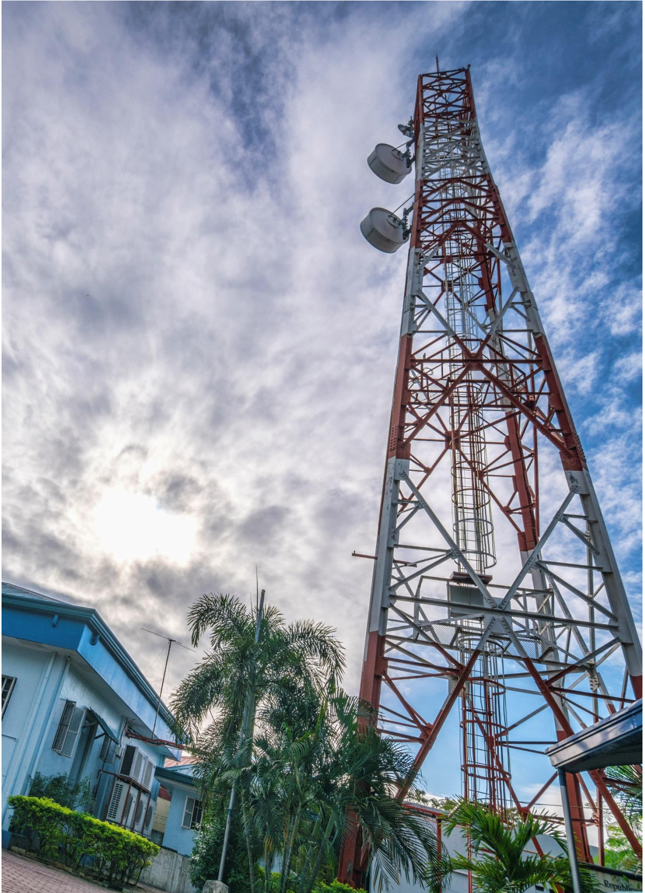
The PRFFWC Telemetry Tower located in the City of San Fernando, Pampanga
