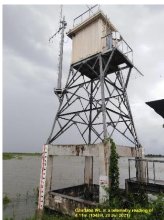
Pic 2 Validation of Candaba WL telemetry reading at 4.11m (1048H, 28 Jul 2021)
