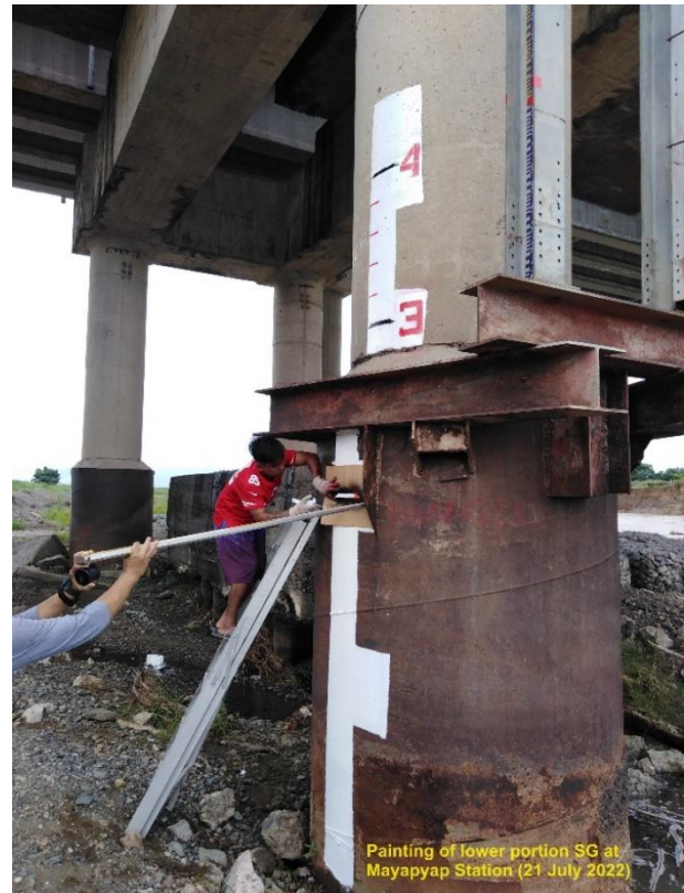
Pic 8 Extending the SG at the lower portion of Mayapyap stream gaging station by painting on the bridge's pier at Bgy. Valdefuente, Cabanatuan City
