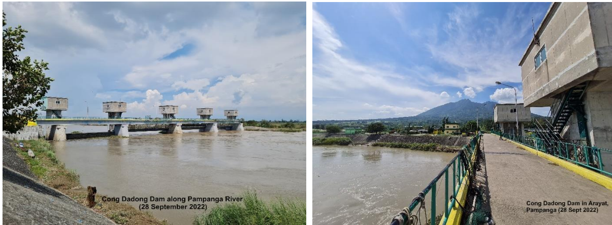
Pic 3 Cong Dadong Dam along the Pampanga River is an irrigation dam and about 2.5 kms upstream of the Arayat Telemetry station which is at the RB of the San Agustin Bridge; the said dam had, at times, affected the flows at Arayat stream gaging station.
