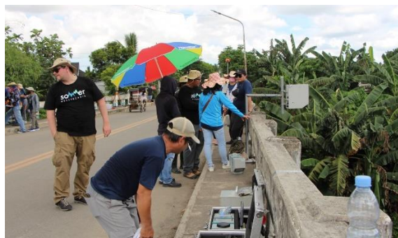
A set-up of Radar Profiler (RP30 and RQ 30) and other instruments at the upstream side of the measuring bridge.
